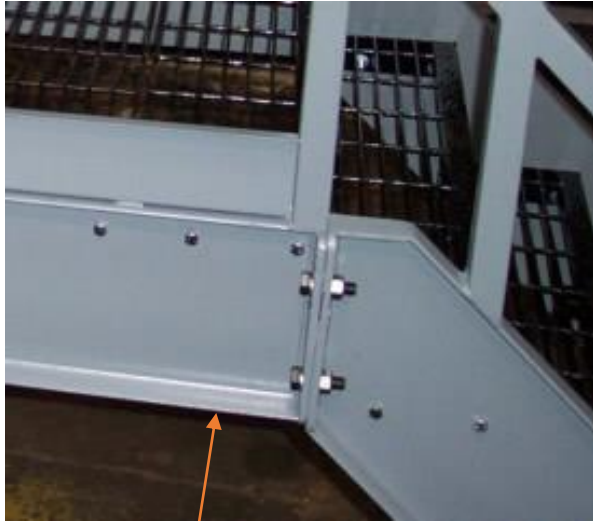
Tek Angle Clip under Extension Channel Bottom Flange
